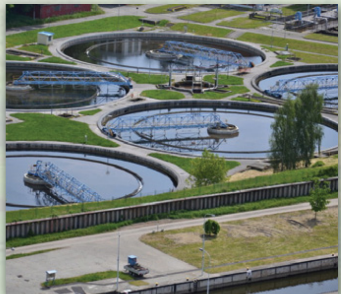
Aerial view of sewage water treatment plant. (Stock image) Photo Credit: josefkubes / Fotolia
